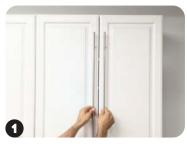
Place hardware (measure as needed) to find position you like; mark bottom hole location with pencil.
