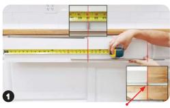
Line up center on one end of hardware hole with edge of drawer front, then measure from opposite end of drawer to the center of the second hardware hole.
