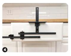
Set the Sliding End Stop to half of the drawer width measurement from Step 3.
