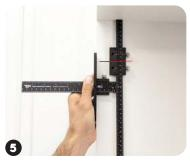
Place two Sliding Drill Guides side by side to achieve 32mm spacing. Position tool with Large Stop and T-square firmly against cabinet surface. Adjust Sliding Drill Guide centers to mark and tighten. Drill first set of hinge plate holes.
