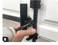
Hold securely and drill through fixed center bushing for bottom hole.
