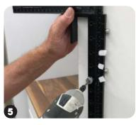
Mark your holes with tape for reference, and drill first set of shelf pin holes.
