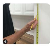
Measure and mark desired location of center hole to be drilled (we are drilling in sets of three).
