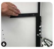
Remove Large Stop and press Thumb Screws against back panel then drill.
