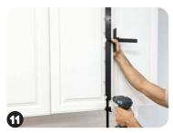
Flip tool to its reverse side, place on opposite door and repeat drilling.
