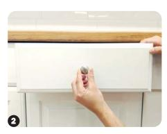
Place hardware (measure as needed) to find position you like, then mark hole location with pencil (We are centering on width and height).
