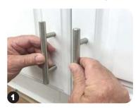
Place hardware (measure as needed) to find position you like; mark bottom hole location.
