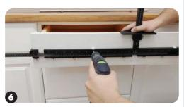
Hold stops firmly against top and side of drawer. Drill through marked holes and install hardware.
