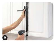
Hold both stops firmly against door and drill bottom hole.
