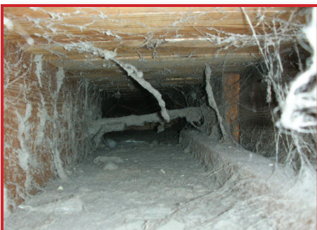
Inspection of hard-to-reach and hard-to-see areas
