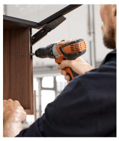
Lift Mechanism Adjustment From the front, adjust the lift mechanism precisely to the weight of the door, preferably with a cordless screwdriver.
